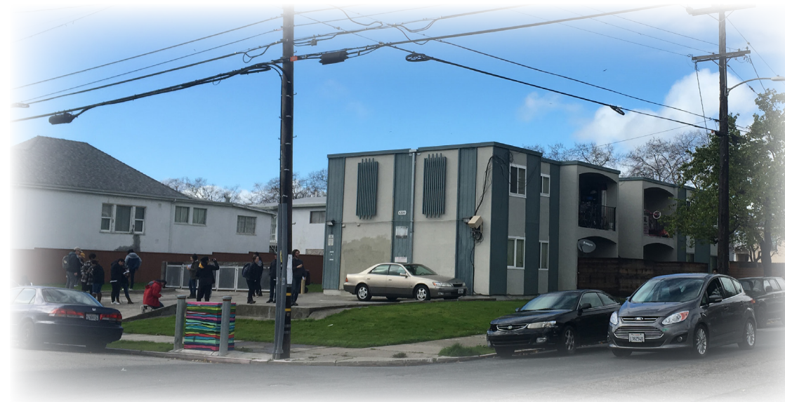
Photo 1.3 Front Perspective of Building
