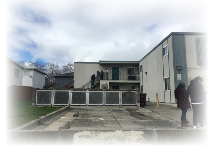
Photo 1.2 Looking lot and trash pick-up from front of building
